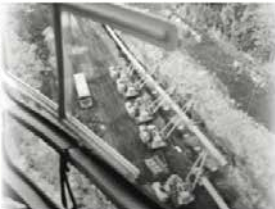
CAT Pipelayers on TransCanada Pipelines Right of Way (ROW) Northeastern Ontario 48" Gas Mainline (Circa 1993).
