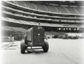
Supplier of a Lincoln Welder for the Skydome build (circa 1989). Ellis Don General Contractor.
