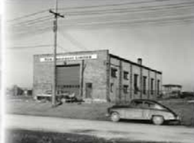
Hub Equipment Branch in Scarborough, Ontario (circa 1957).
